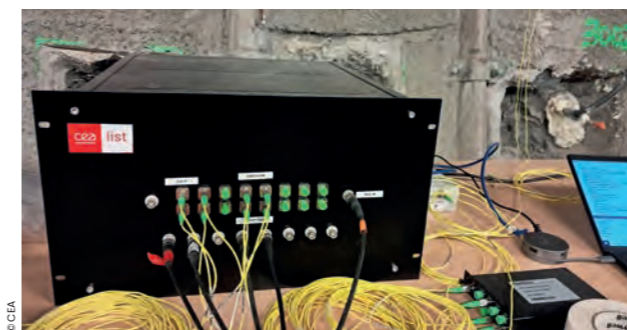
Figure 1: Optogéro measurement system deployed at Bure
